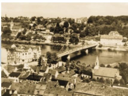
1777 BUTTING foundation in Crossen/ Oder as coppersmith's
